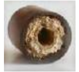
Lime scale build-up in copper pipe
